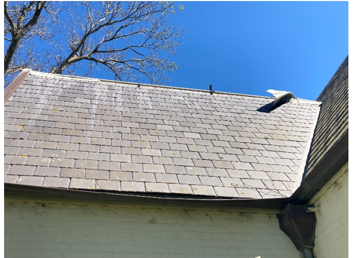
The solid lead roof ridge capping of south storage wing of the St George's Old School Hall wing was blown off
