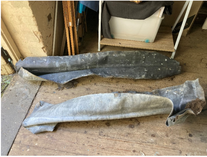
The solid lead roof ridge capping of south storage wing of the St George's Old School Hall wing was blown off
